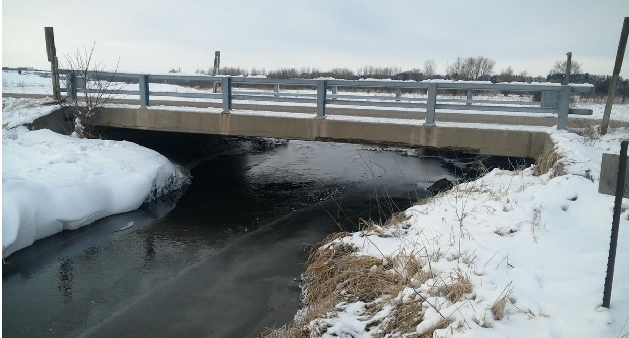
Figure 9. White Crossing Road Bridge span is 40 feet
