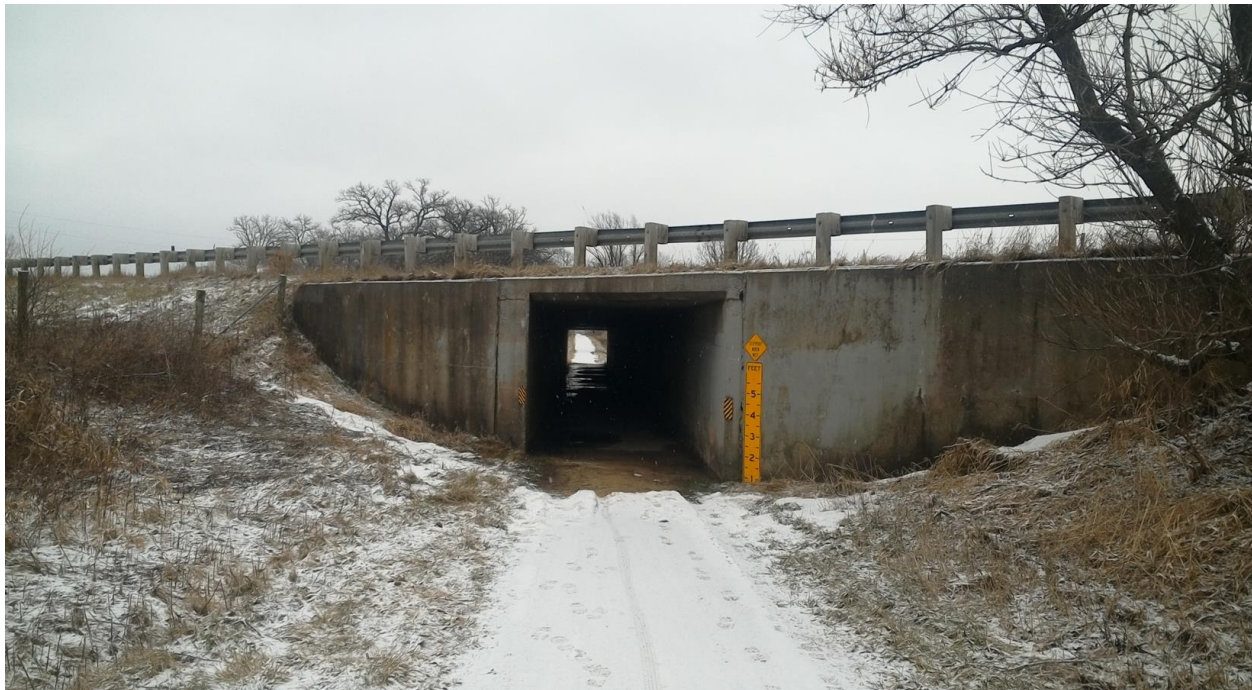
Figure 13. Military Ridge State Trail box culvert under the USH 18/151 Crossing
