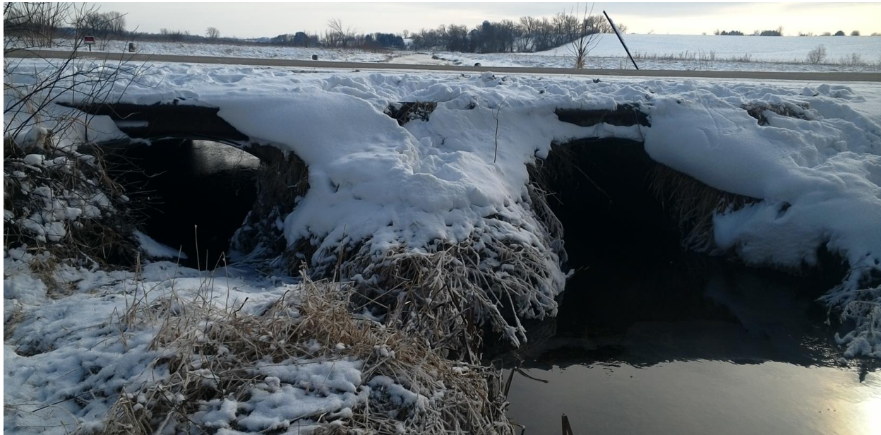
Figure 10. White Crossing Road 48-inch by 66-inch culverts
