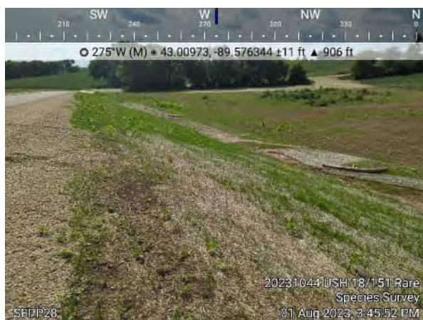
Photo #23 SFPP28, view west of road shoulder of recently constructed extension of Country View Road
