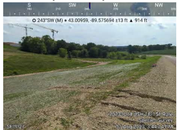
Photo #22 SFPP 27, view southwest of road shoulder of recently constructed extension of Country View Road
